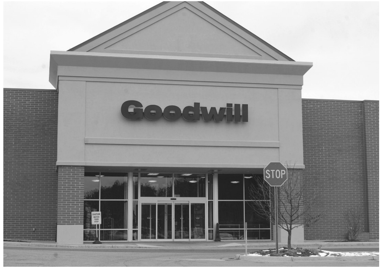
The 6,700 square foot Goodwill Retail and Donation Center in Petoskey is located at 1600 Anderson Road. PHOTO BY DAVE BARAGREY
